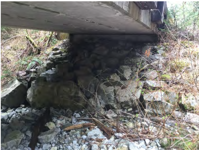
Right Bank Abutment when facing downstream
