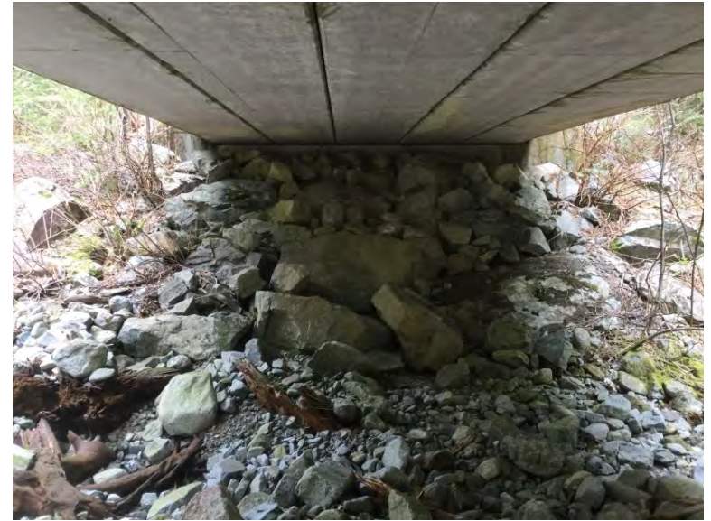
Left Bank Abutment when facing downstream
